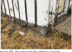
Image 02 - No adequate foundation support
