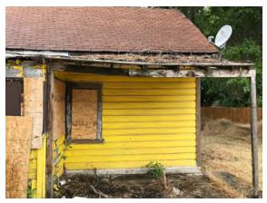
Image 04 - Rotting wood structure with roof on the verge of collapse
