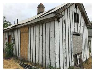
Image 01 - Rotting wood structure
