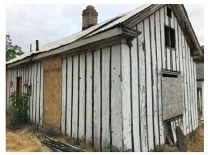
Image 01 - Rotting wood structure
