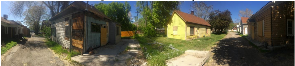
Bishop Place Panoramic View (Looking North at Center of Frame)
