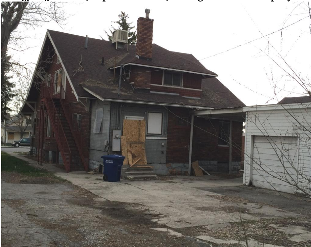
432 N 300 West Rear View
